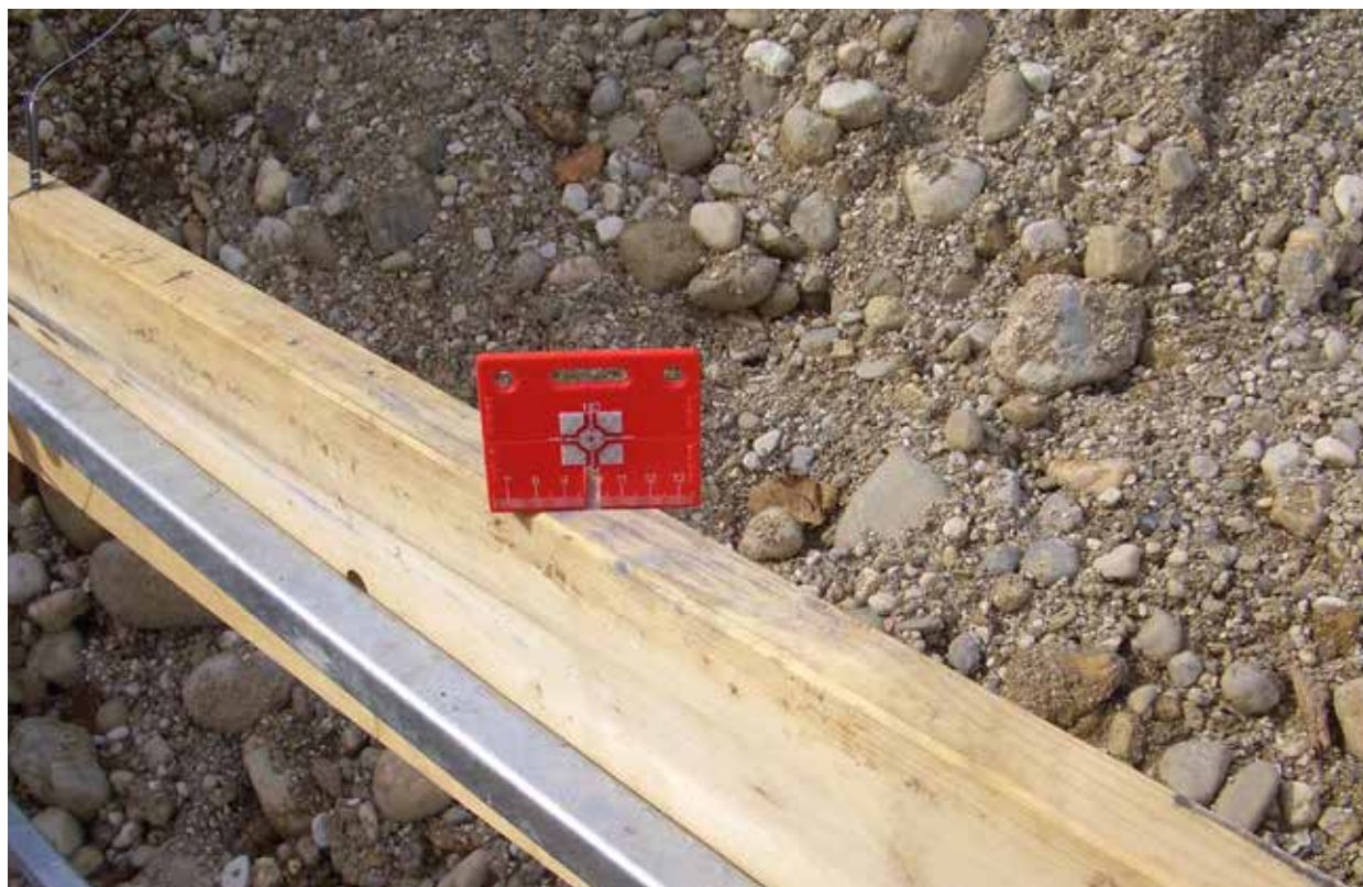
RS95 – Stake out work on the batter board.
