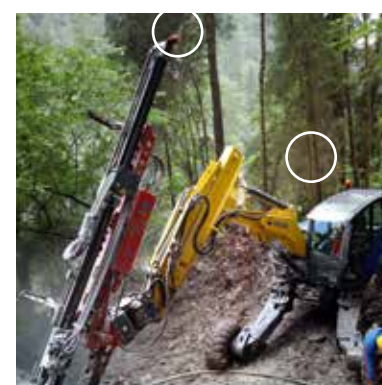
Example of the use of RS193rM as a fixed point on different surfaces and for the exact alignment of the drill carriage.
